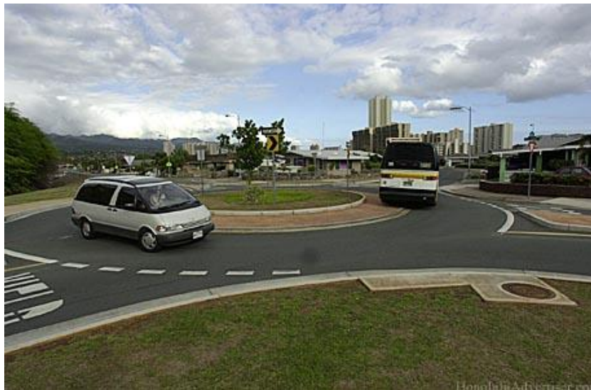
Figure 5 - Ala Napunani St/Likini St Roundabout example
